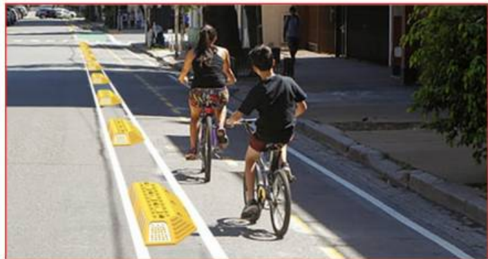
It is anchored to the floor with 7 nails of \frac{1}{2} " x 10" and epoxy resin
