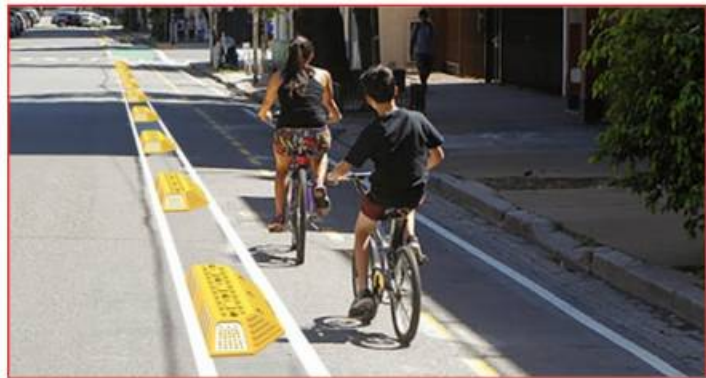
It is anchored to the floor with 7 nails of 1/2" x 10" and epoxy resin
