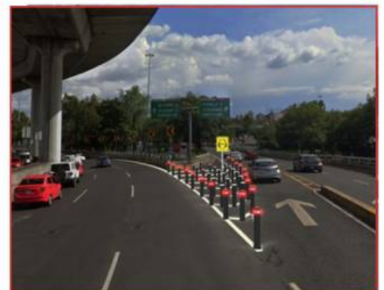
Robust and flexible inner bollards. Reboundable arrow sign for impacts.
